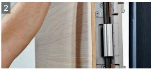
The door leaf is connected to the frame. Now, the hinges are inserted into the frame recess. An assembly dolly can serve as an aid or assembly cushions, wedges, etc. can be used.
